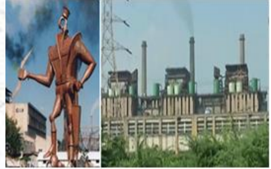
Industrial visit to Nashik Thermal Power Station, Eklahare on 4.9.2024.
